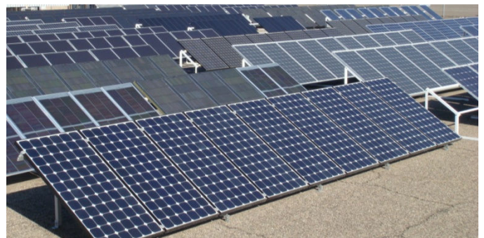
Fig. 2. The 2 kW system used in this study is the front 9 modules.
